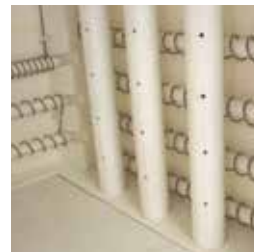
Perforated ceramic tubes for injecting preheated fresh air
